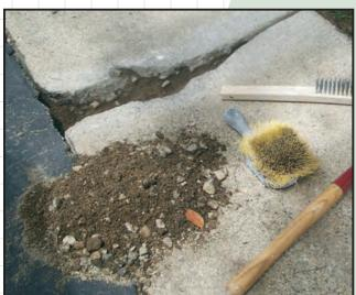
Duct tape, brooms and paint brushes are excellent tools in the application of MG-KRETE<sup>TM</sup>.
