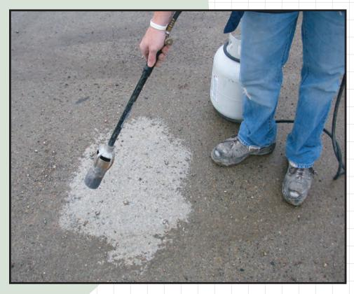
continue to be heated for approximately one hour to ensure a reasonable cure. Good ventilation is most important in small enclosed areas. The ammonia gas given off during cure will pose a problem if not well ventilated.
