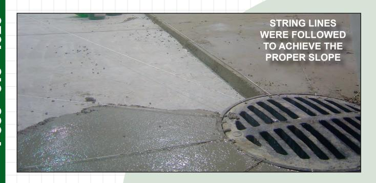
MG-KRETE<sup>TM</sup> is very effective when it comes to re-sloping concrete surfaces. Water pooling in garages is usually the biggest problem. To repair sloping issues one needs to acquire the desired slope. This can be done with the use of a simple string line, laser level, level or screed. Rebuild and fill any deep areas with MG-KRETE<sup>TM</sup> first. Once the desired slope is determined you
