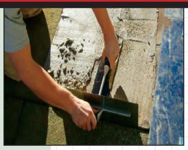
When rebuilding edges be sure to make your mix dry enough so the MG-KRETE<sup>TM</sup> does not slump.
